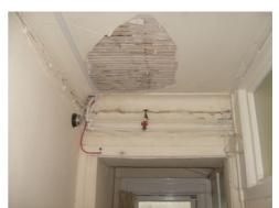
Above are some parts of the kitchen ceiling which have been damaged by a leaking roof and dampness. Several other ceilings and walls in the monastery are also damaged.
